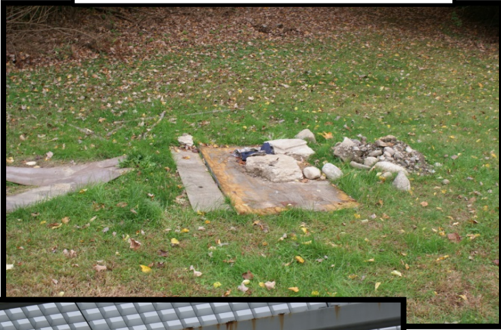
Old septic system distribution box
