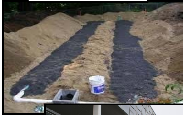
New septic system Installation
