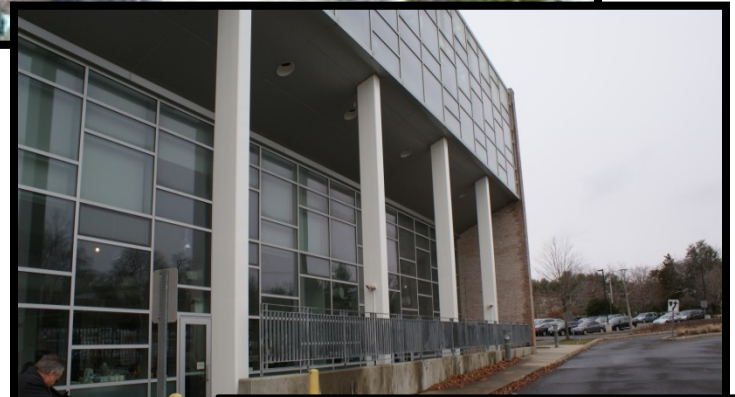
New exterior structural steel freshly repaired and painted
